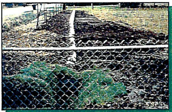
Figure 4-14: Pipeline replacing contaminated ditch.
