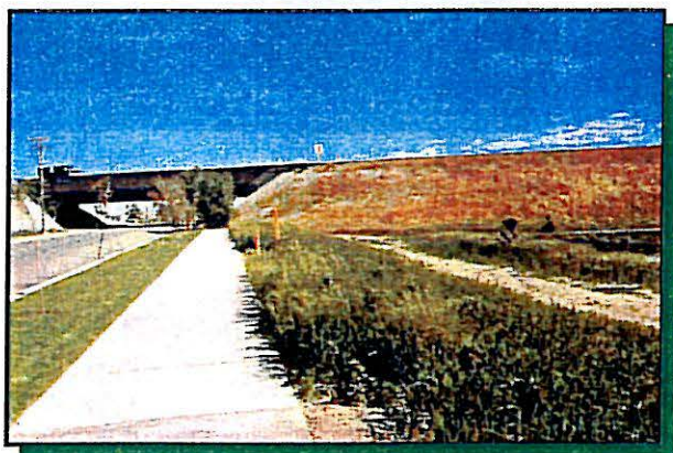
Figure 4-5: Contaminated soil could be used as fill for an overpass.
