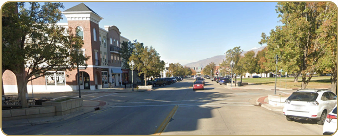
Example of intersection bulb outs and on-street parking (street view) - Bountiful, UT
