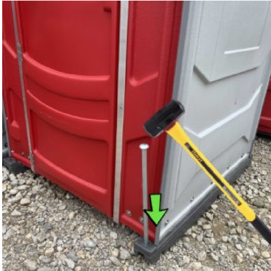
Figure 28: Photo showing staking of portable toilets to secure from tipping
