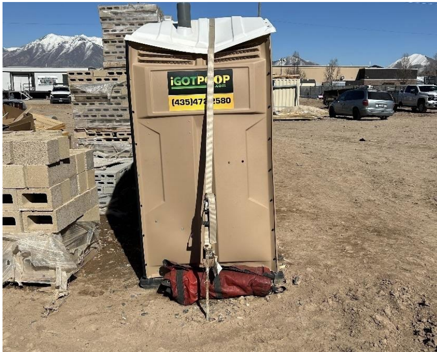
Figure 29: Photo showing portable toilet secured with tie-down straps
